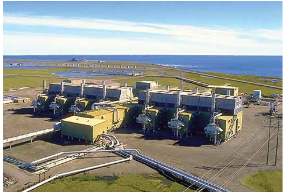
Prudhoe Central Compression Plant.
