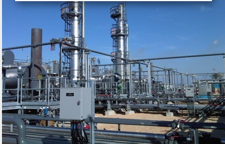
Eagle Ford Condensate Stabilization
