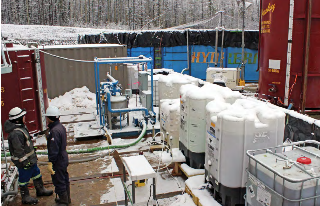
Water treatment chemical storage area
