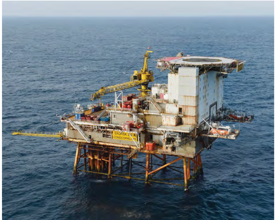
A view of the Ekofisk 2/4 A platform, part of the decommissioning efforts in the southern Norwegian North Sea. Ekofisk 2/4 A was the first permanent production platform on the Norwegian Continental Shelf. It was in active service from 1974 to 2013. In Norway, ConocoPhillips is optimizing existing P&A technologies and processes and testing step-change technology projects. Improved traditional milling operations, the proven “PWC” (perforating, wash and cement) method and the use of formation as P&A barriers have been of particular value.
